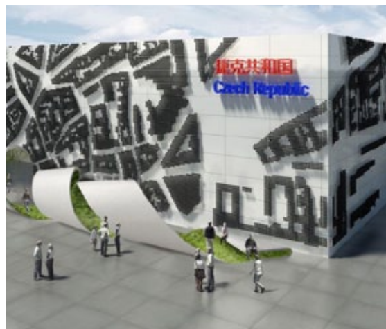
Exterior of the Czech pavilion during daytime. The facade is created from Czech hockey pucks. (source: Office of the general commissioner of Czech participation on EXPO 2010)
